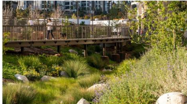
Integrated Stormwater / Rain Garden
