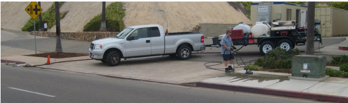
Set up (Observe slope of street, block storm drains, test vacuum)
